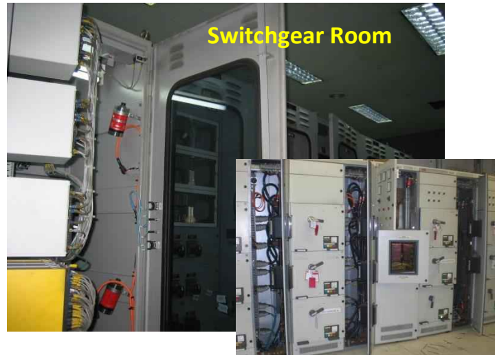
Electricity Generating Authority of Thailand (EGAT) Thailand, 2012
